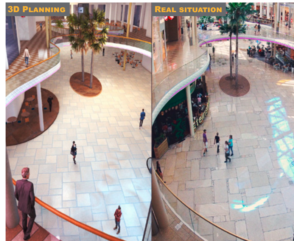
"What we plan is what you get" – 3D planning and real situation compared
